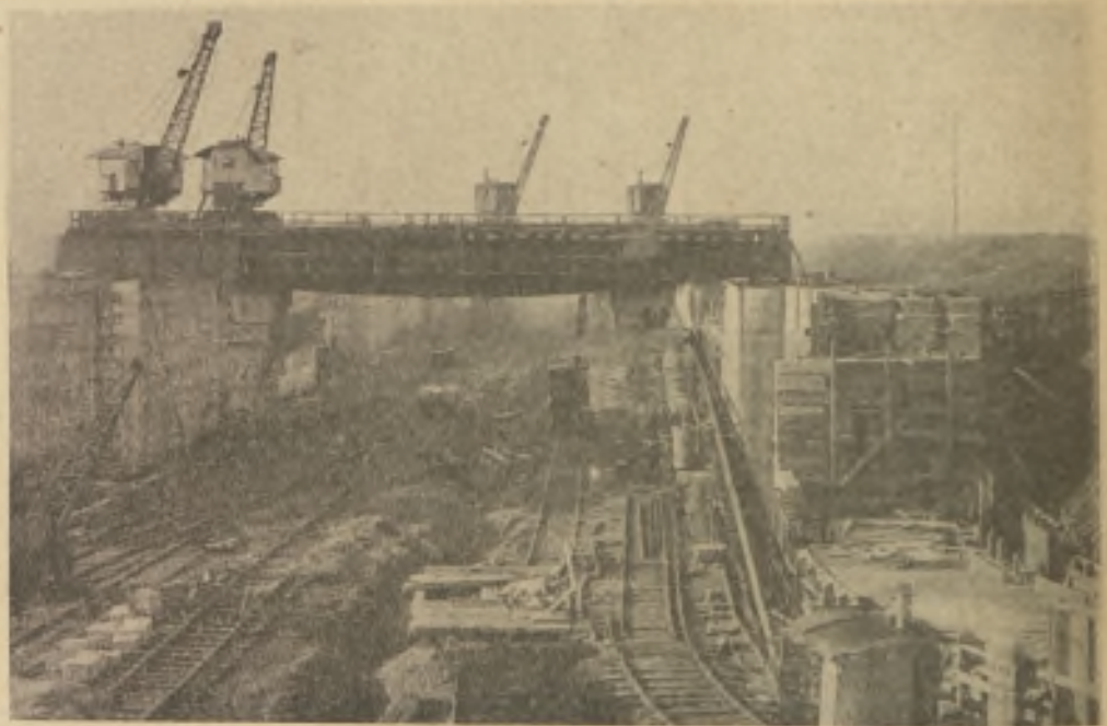
King George V. Dock's great lock under construction.
