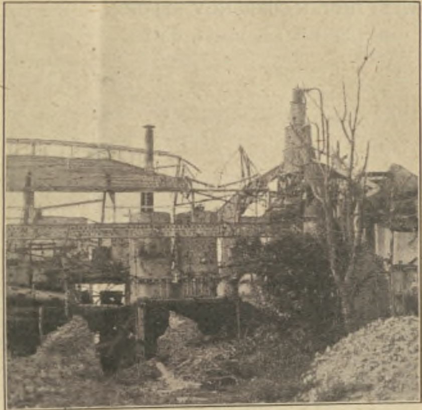
A WRECKED FACTORY IN FRANCE.
