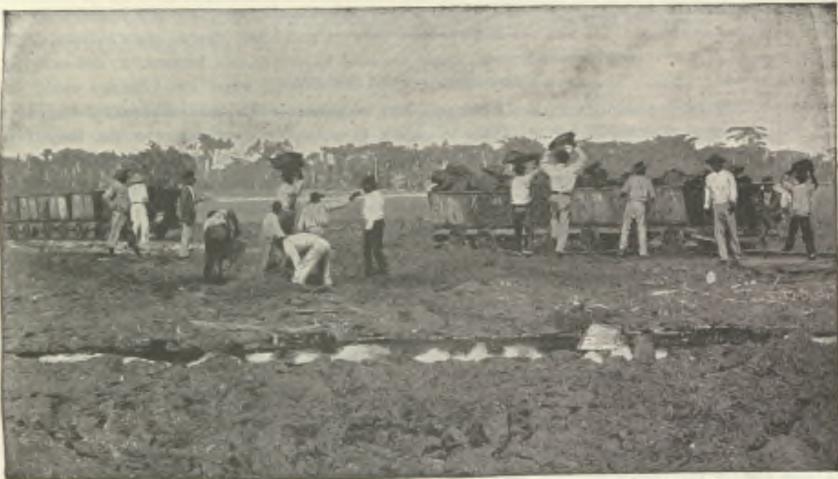
Digging and Loading Pitch at the Pitch Lake, Trinidad.
