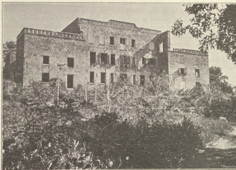
The dismantled Bath House Hotel, Nevis.
