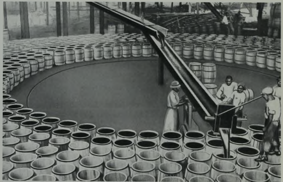
A Pouring Circle. Dehydrated asphalt being casked for shipment
