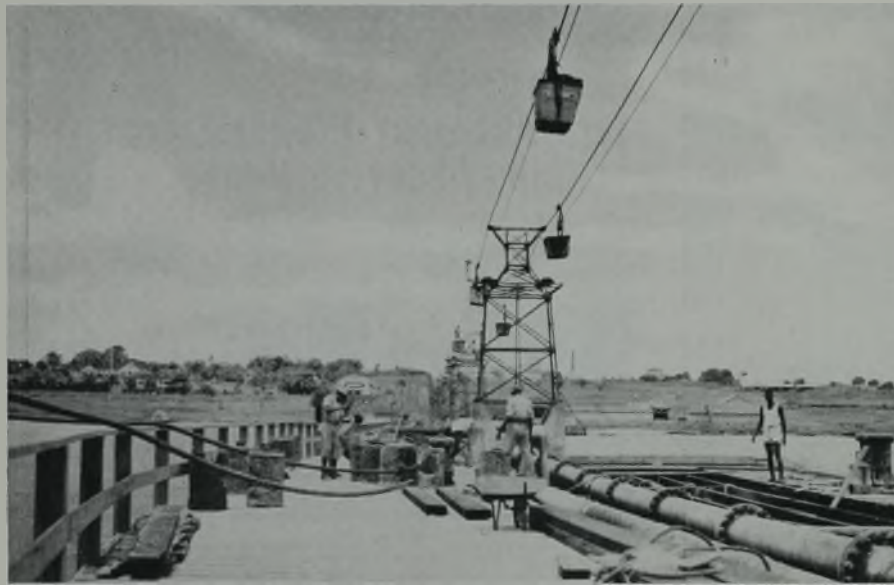
Overhead cableway carrying crude and refined asphalt to the ships
