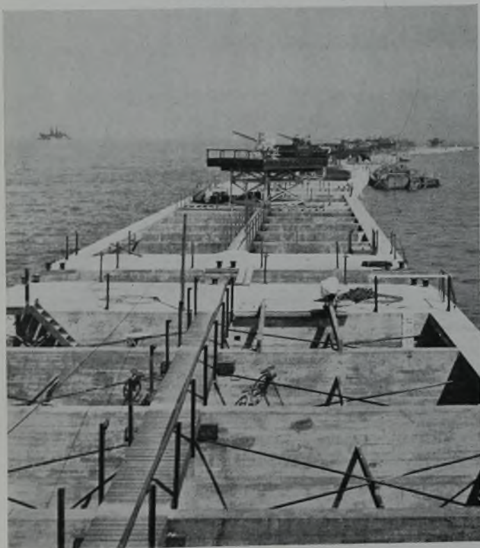
CONCRETE CAISSONS FORM DEEP WATER BREAKWATER
