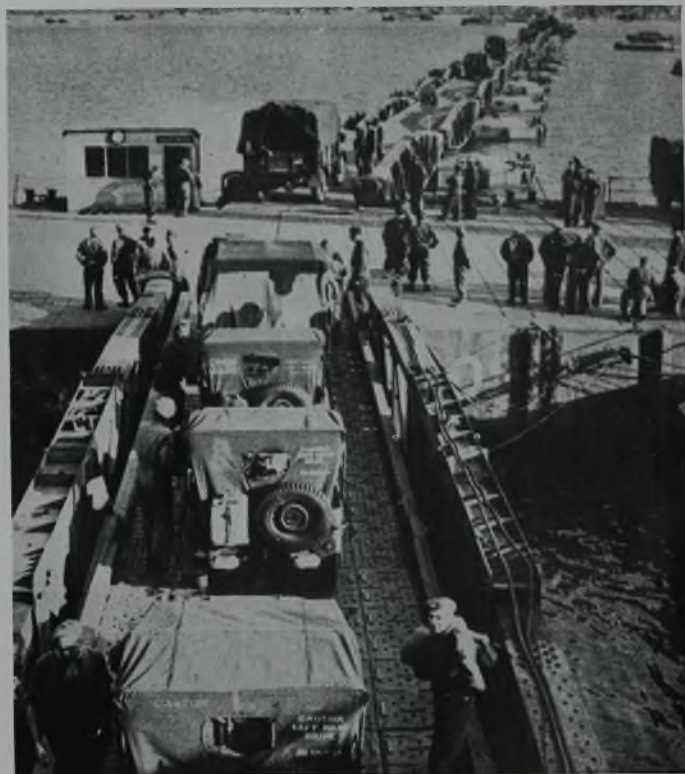
A BUSY SCENE ON ONE OF THE PIERS
