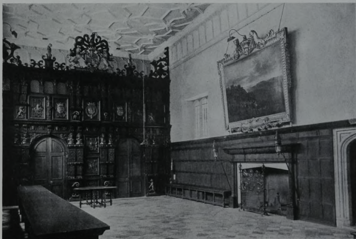
THE NORTH END OF THE MAIN HALL
