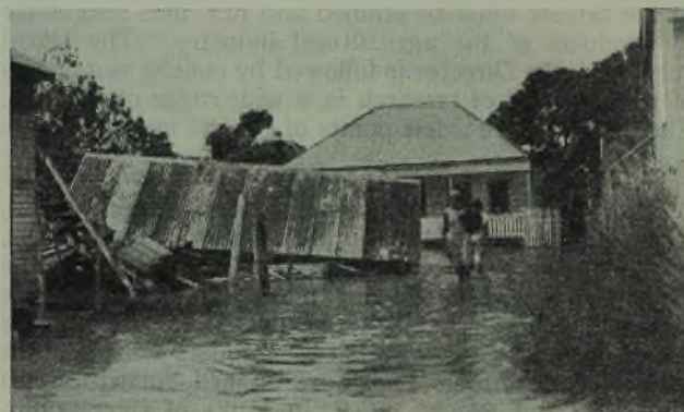
Damage in Main Street, Stann Creek
