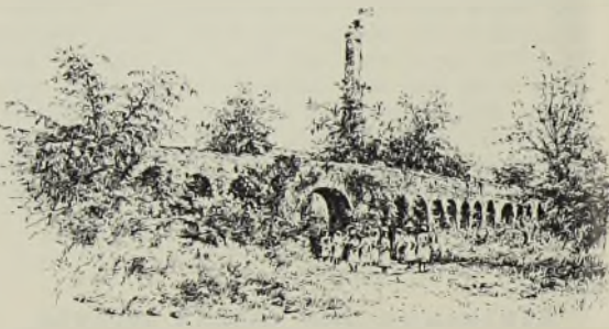
Fort William Aqueduct.
