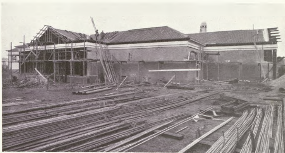
Nearing Completion : The Building with the Northern Annexe, on February 7, 1924.
