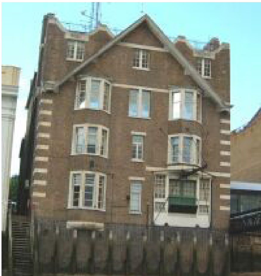
Wapping Police Station as it looks today.
