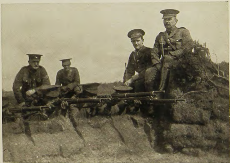
TRENCHES AT WITHNOE CAMP
